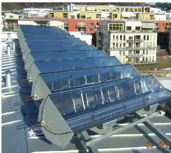
Fig. 1.5. Photograph showing an array of compound parabolic concentrators for PV and Thermal application
